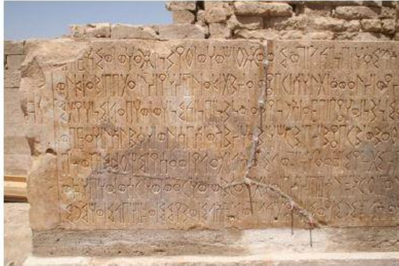
Fig. 5: The closed fissure on the western front side of the stone.
