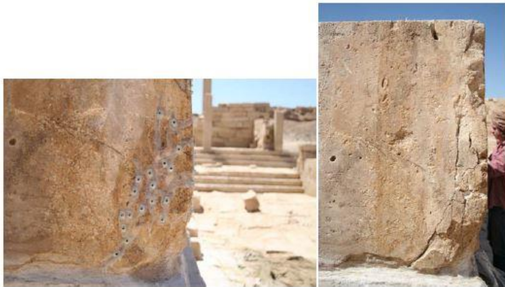
Fig 3: Left: Eastern side of the stone with fissures covered by hot glue. Right: the fissures after fillings with epoxy resin.
