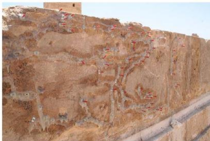
Fig. 4: The large loose part in the middle of the stone covered by hot glue. The injection channels are closed by red caps.
